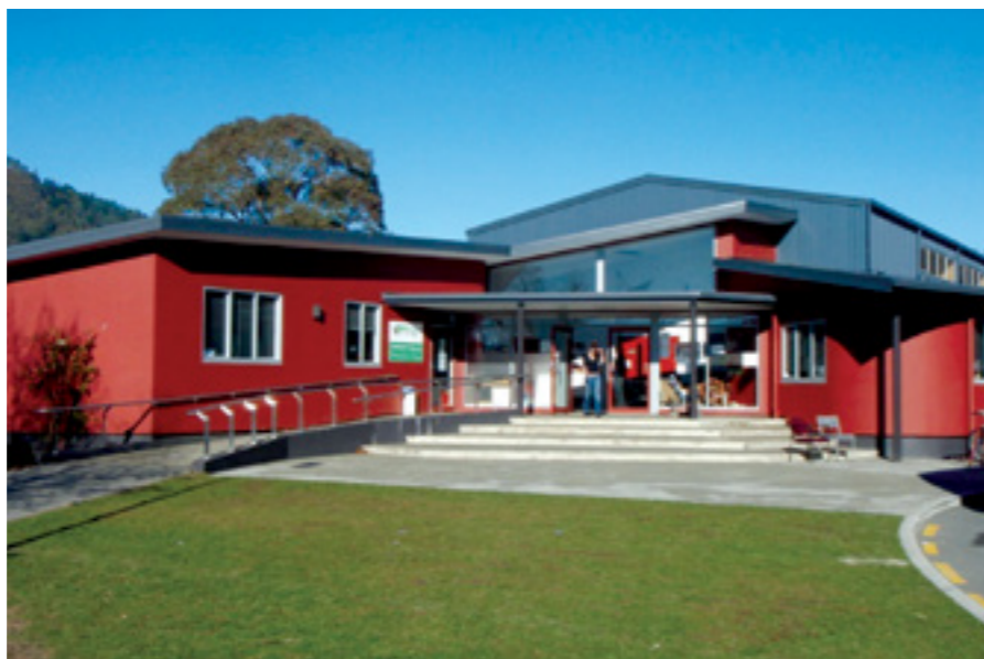
Victory Community Centre is based at Victory Primary School and includes a combined school hall/community hall, a health clinic, shared office space and meeting rooms.
